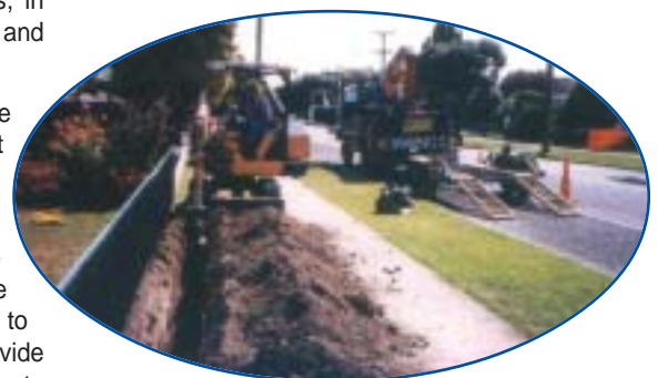
Undergrounding of power lines
